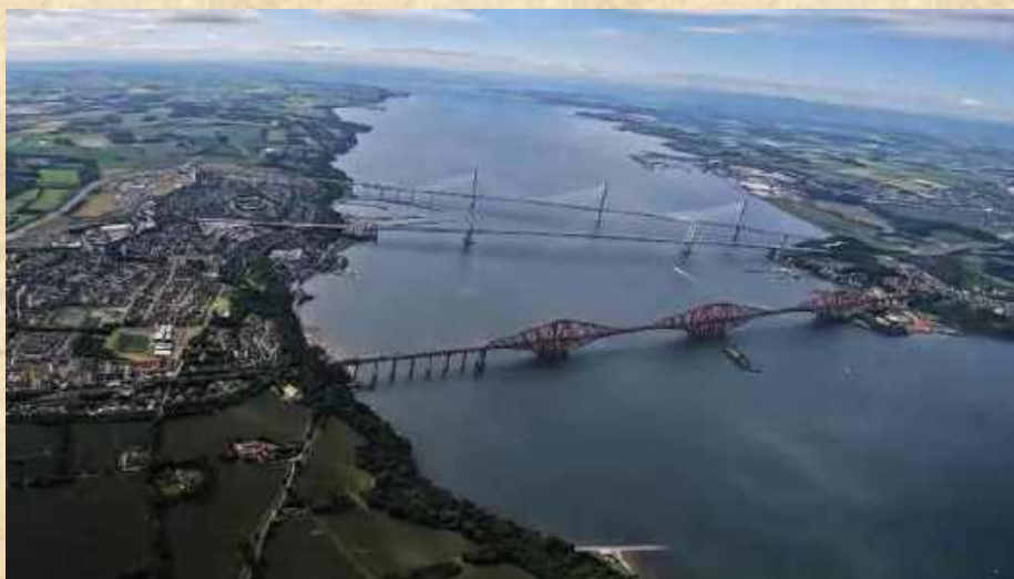
FROM TOP TO BOTTOM – QUEENSFERRY CROSSING, FORTH ROAD BRIDGE, AND FORTH BRIDGE
