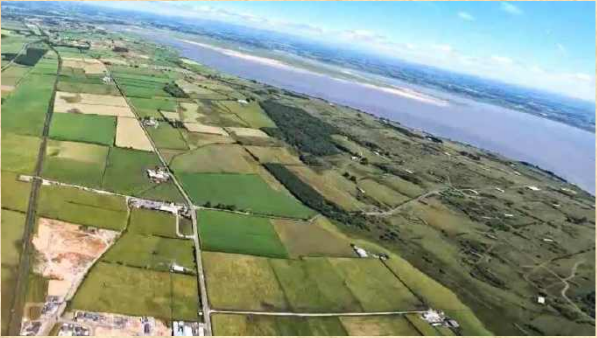
PART OF THE EASTRIGGS ARMAMENT FACTORY, STRETCHING FOR 9 MILES ALONG THE COAST
