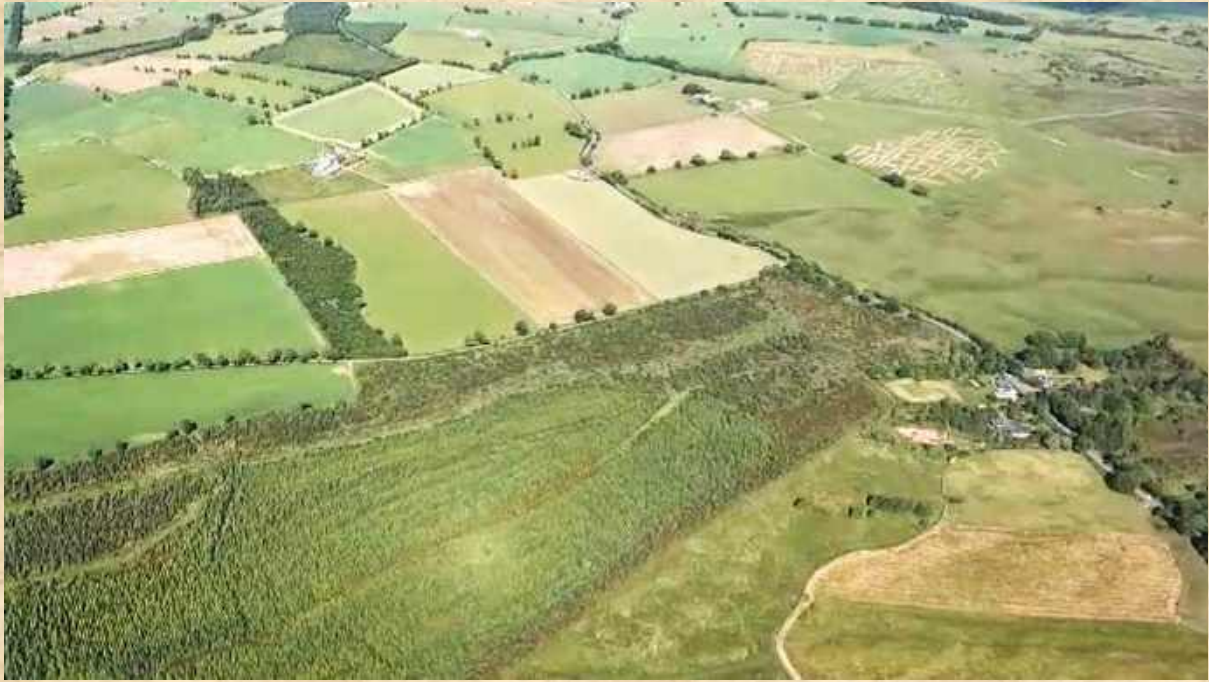
ON THE FAR RIGHT OF THE PLANTATION CAN BE SEEN THE SQUARE KAIMS FORTLET FOUNDATIONS
