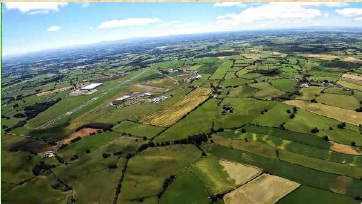
CARLISLE LAKE DISTRICT AIRPORT WITH THE WALL ROUTE FOLLOWING TREE LINE TO ITS RIGHT
