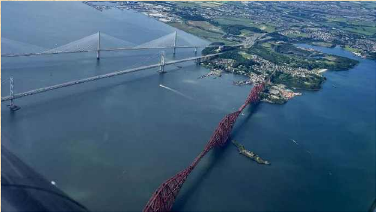
'THE BRIDGE'S VRP
