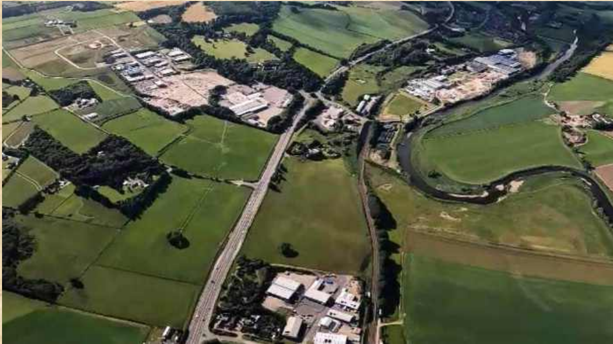
SITE OF THE TWO MARCHING CAMPS AT KINTORE
